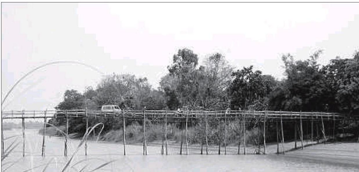
■ This bridge is the only way of communication for villages between East and West Midnapore.
